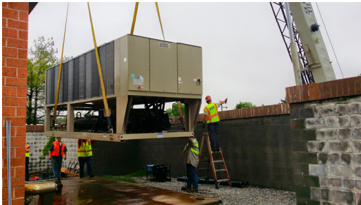
Daikin Chiller Replacement Project Quantico VA
