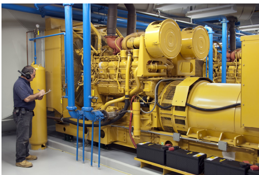
Standby Emergency Generators PM Service
